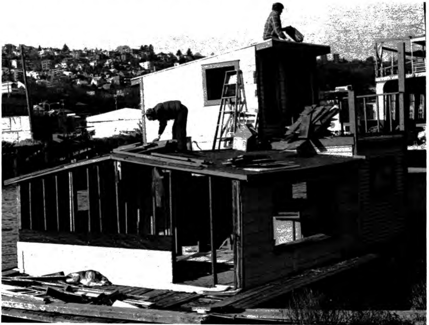
Robert Weppner's floating home, evicted by court order from the James Jessup moorage, 3125 Fairview E., is shown being demolished for salvage. Weppner sold it for $1.00 with the understanding that the new owner would remove it from the illegal occupancy in a State Waterway where it was abandoned by the sheriff's department in carrying out the court order. The new owner was also unable to find a place to moor it. Prior to eviction the houseboat was appraised at $20,000.00. (Photo by Jonathan Ezekiel.)
